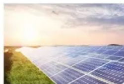
Energy Storage System
